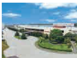
CHINA China Plant (MCC)
